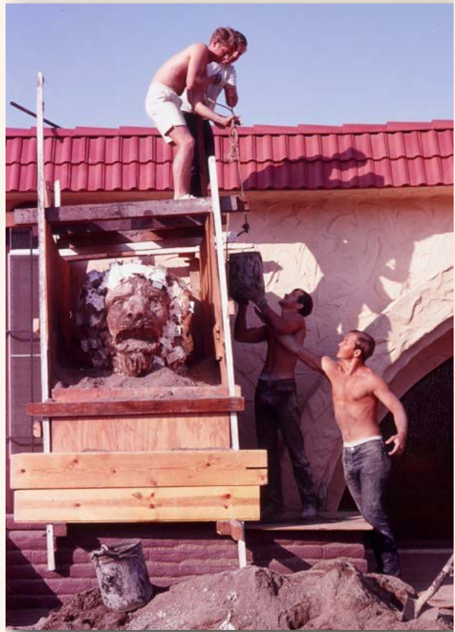
Pouring the Concrete for the Lions
